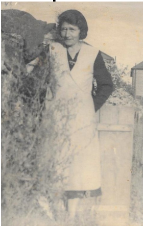
Rose's Mum outside the Anderson shelter in Selbourne Rd
