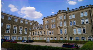
Elim Conference Centre (photo above)
