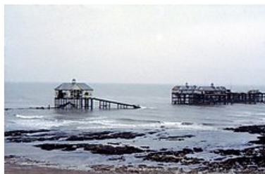
The remains of the pier after the 1978 storm surge
